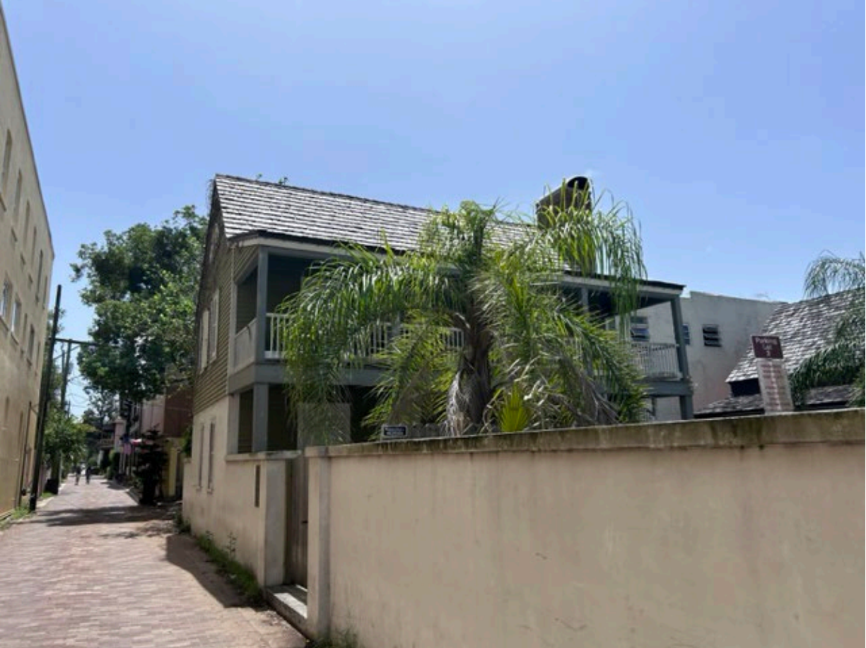
Figure 2. View of the Watson House property looking south on Charlotte Street.
