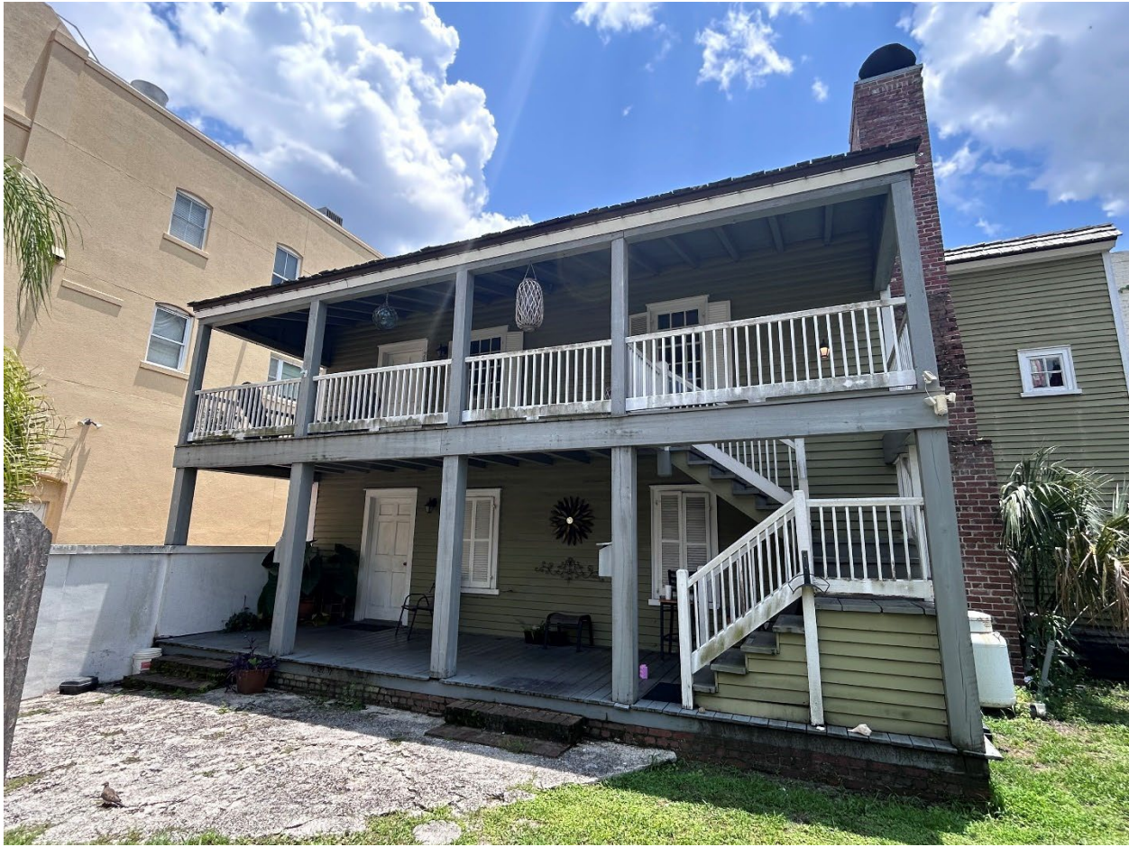
Figure 8. View of the Watson House’s front façade from the yard.
