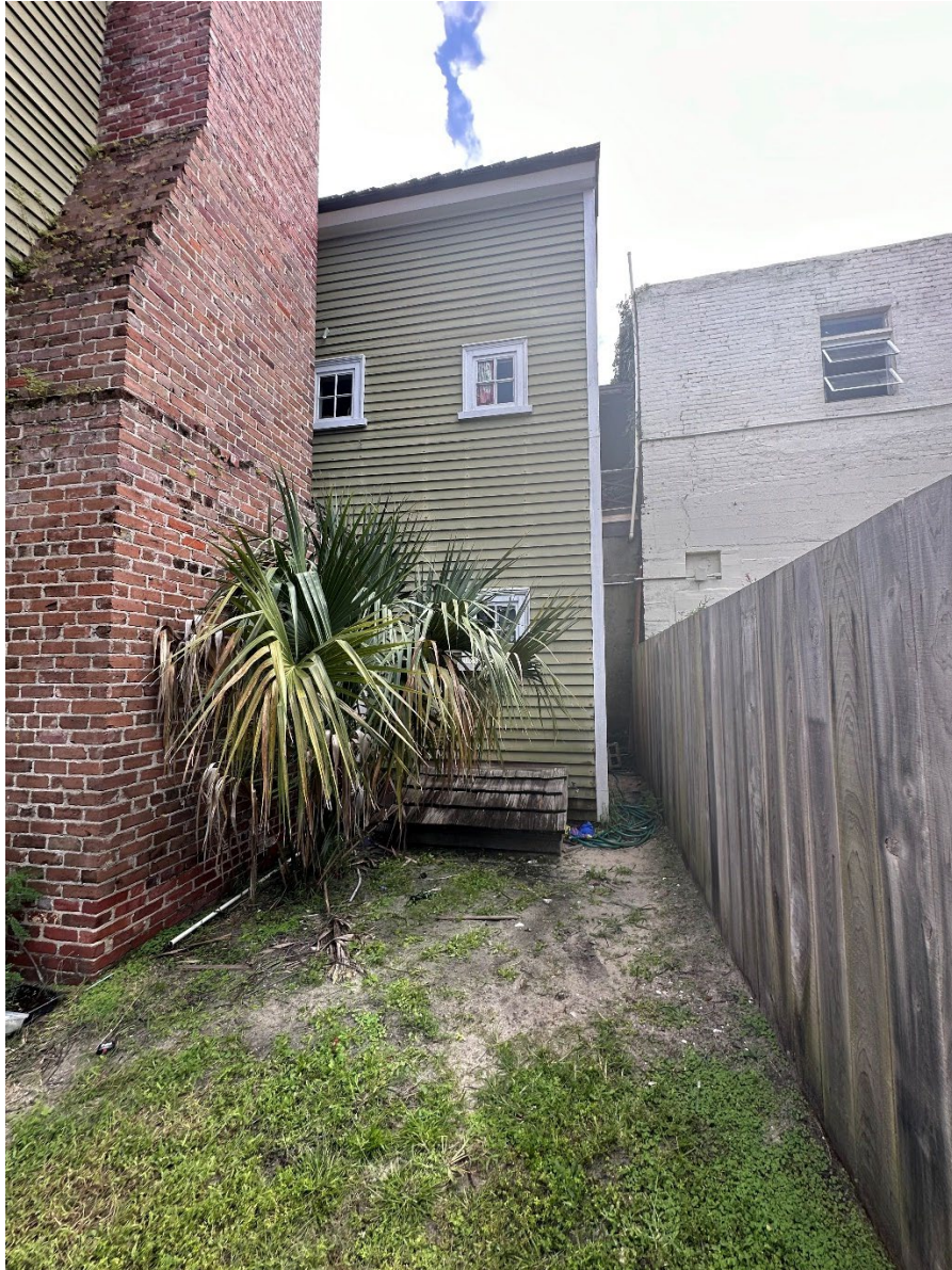
Figure 4. View of the southwest corner of the Watson House.
