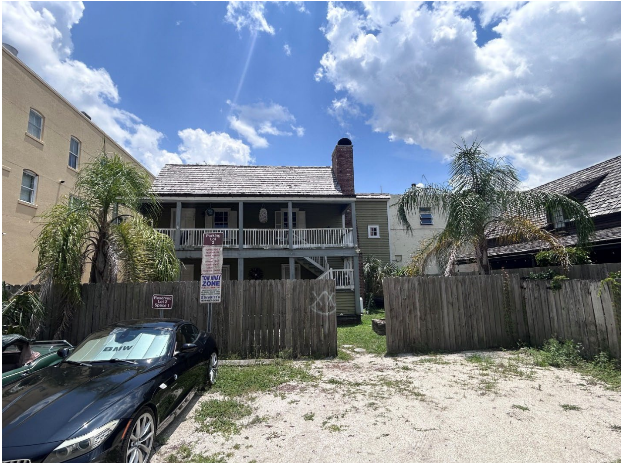
Figure 6. View of the Watson House from the parking lot.
