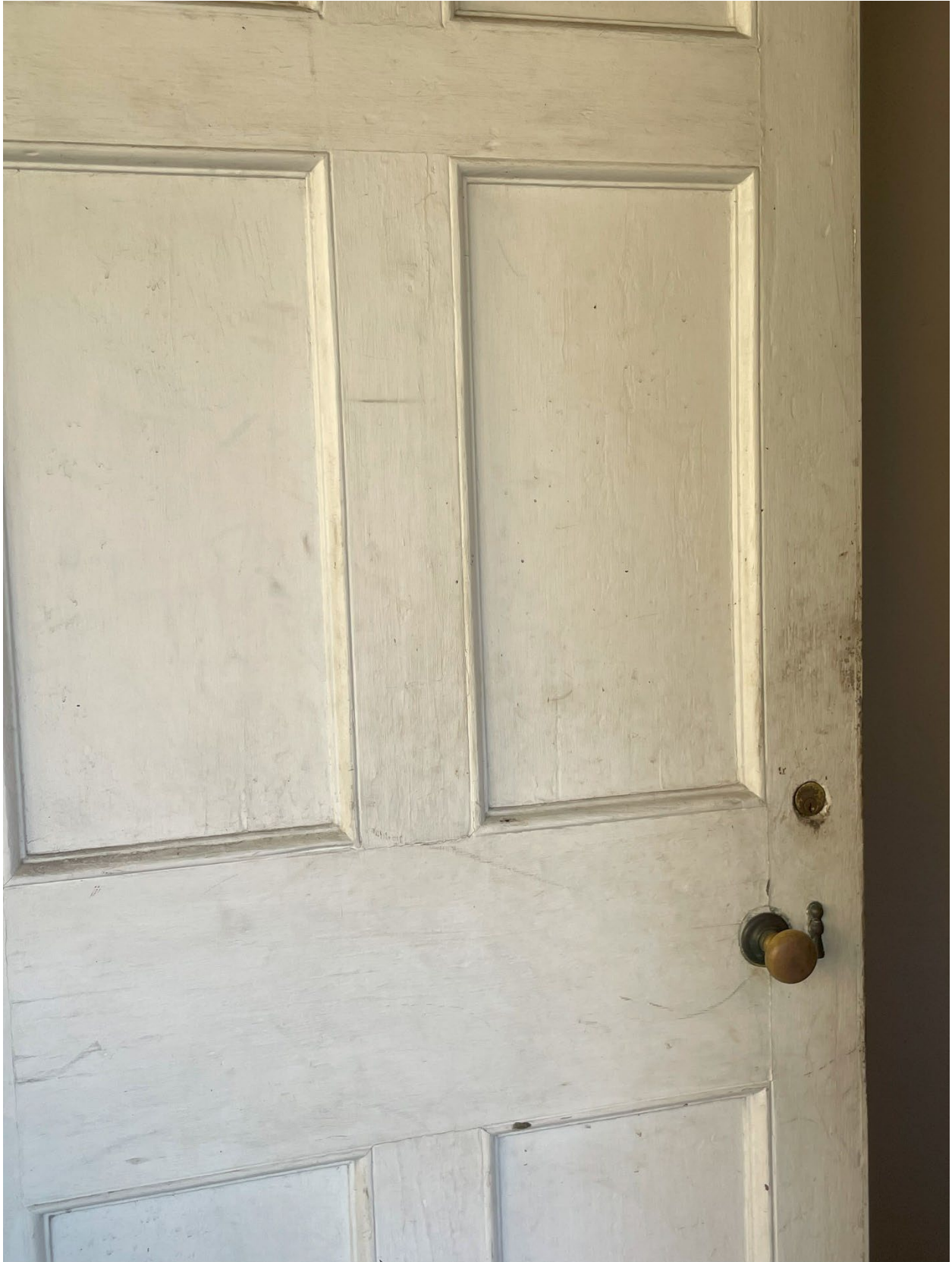
Figure 8. View of the second floor Entrance door.
