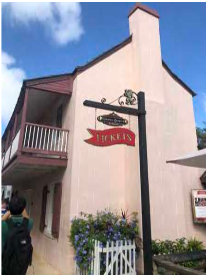
B: West Wing, S facade, looking NE
