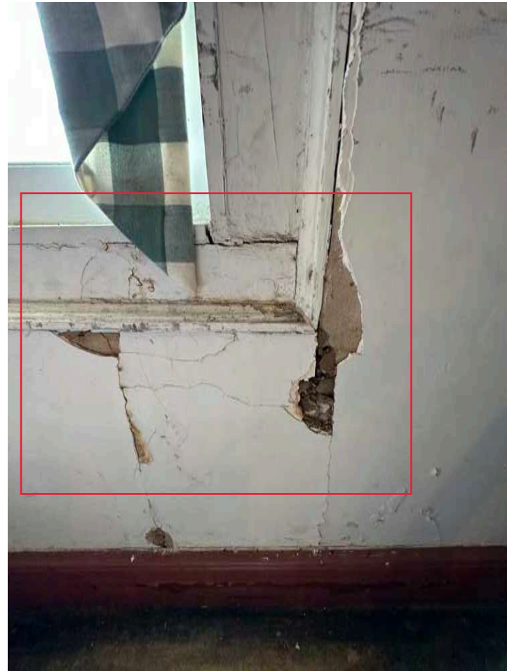
B: Room 207, looking S
