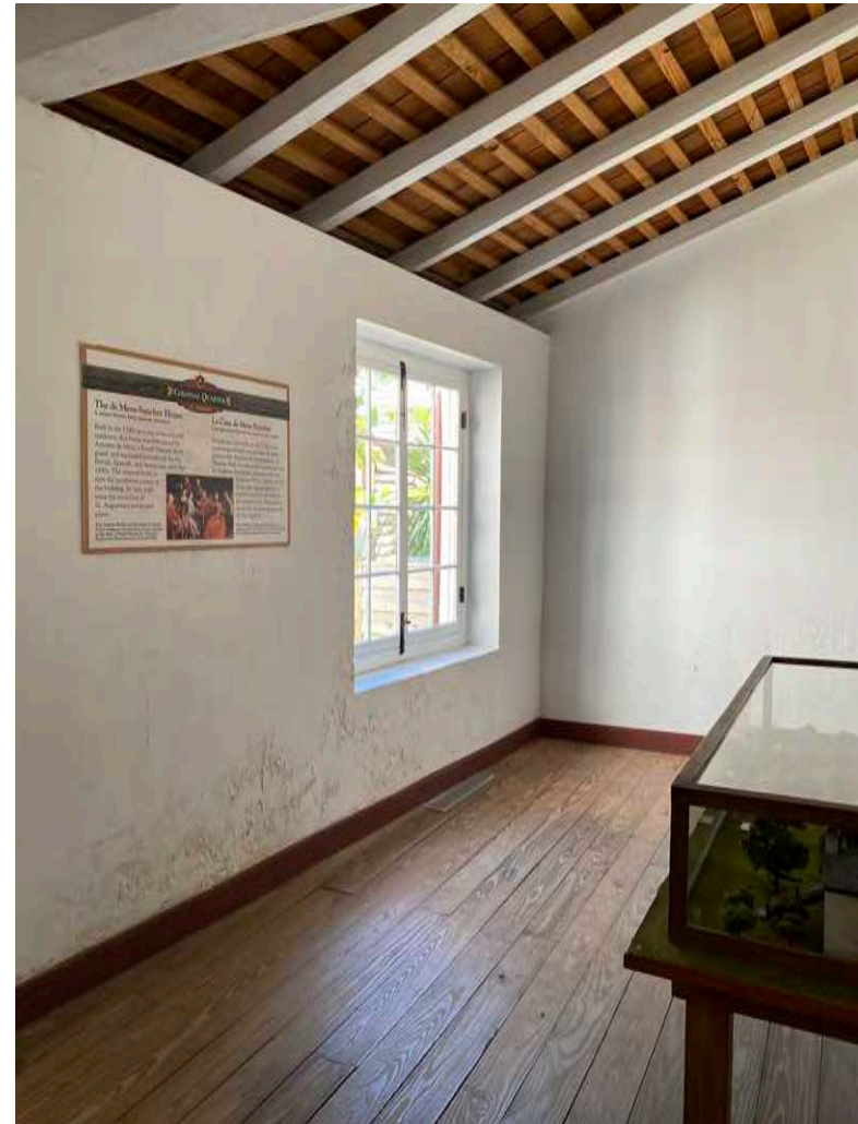
DeMesa- Sanchez House, Room 104, east wall, looking SE, 2020. Photo: Sarah Ryan
