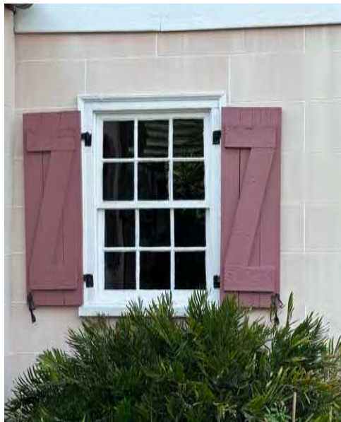
A: East Wing, window 1S3, looking N
