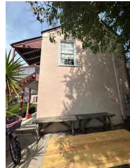
A: East Wing, E facade, looking W
