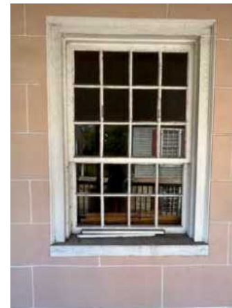
F: West Wing, W facade, looking E
