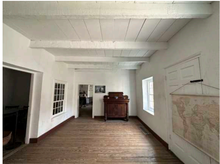
B: Room 107, looking E
