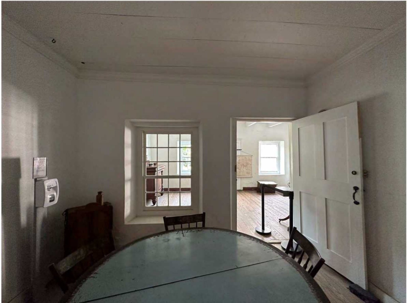
A: Room 108, looking S
