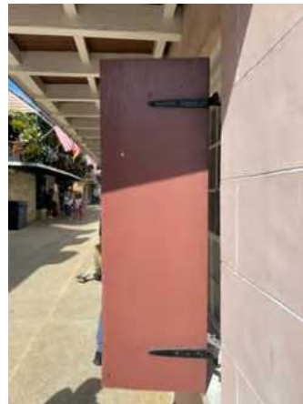
E: West Wing, W facade, looking N
