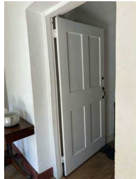
F: Door D9 looking NW
