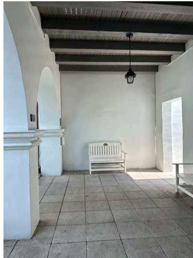
B: East Wing, N facade, looking S Window 2N1, not accessible for viewing
