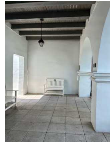
C: East Wing, N facade, looking S.
