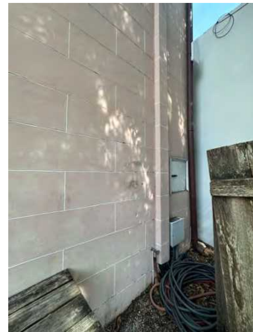
C: East Wing, S facade, looking NW
