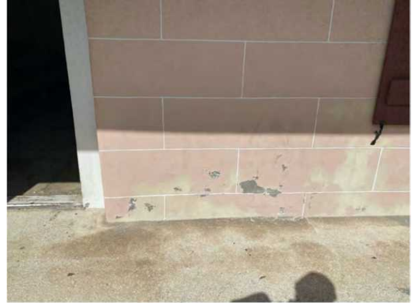
B: East Wing, S facade, looking N and down
