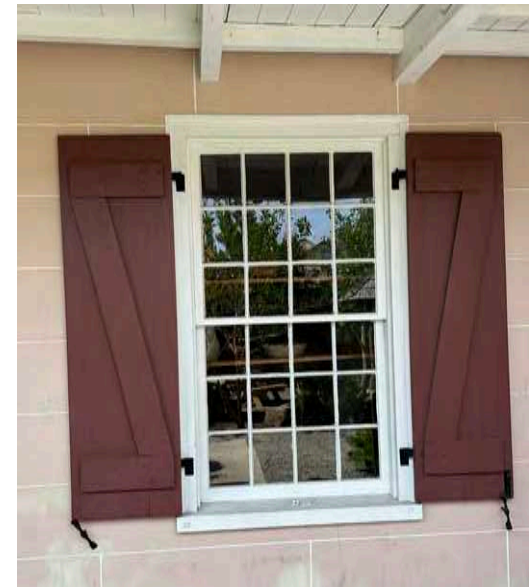
C: East Wing, window 1S1, looking NE
