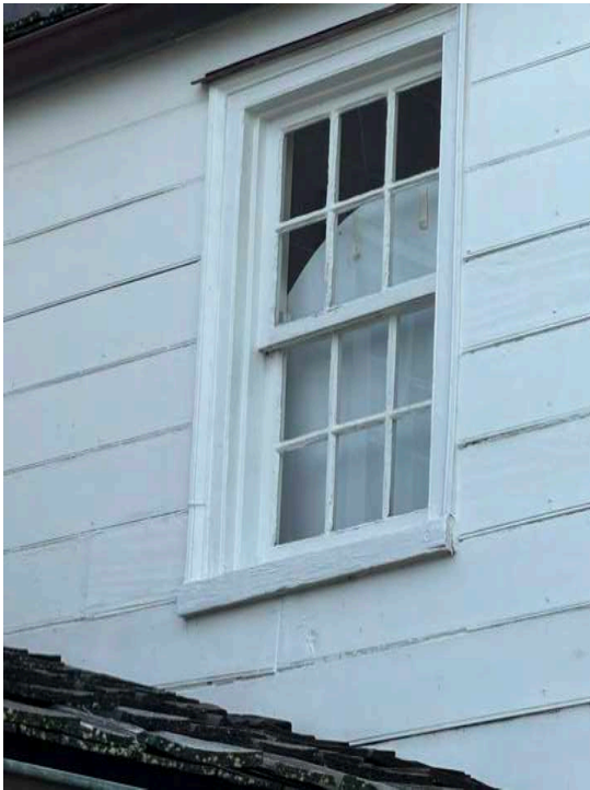
A: East Wing, window 2S5, looking NE and up
