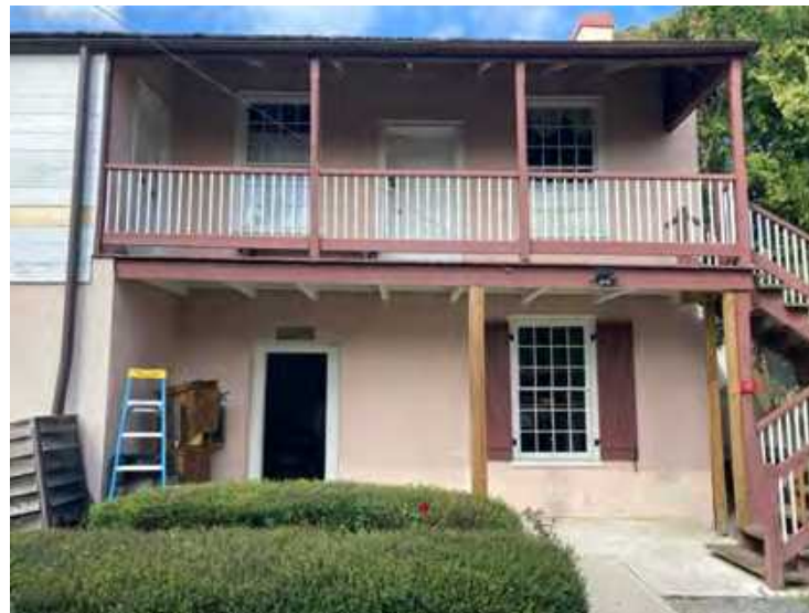
B: East Wing, S facade, looking N
