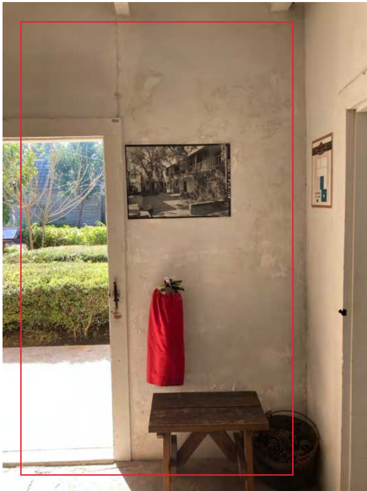
A: Room 110 , looking S
