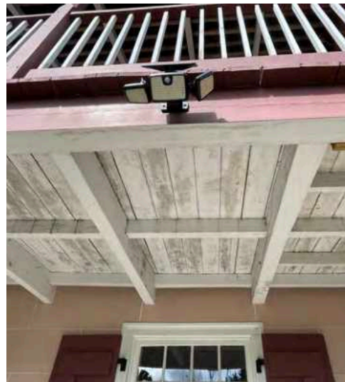
E: East Wing, Loggia, looking N and up
