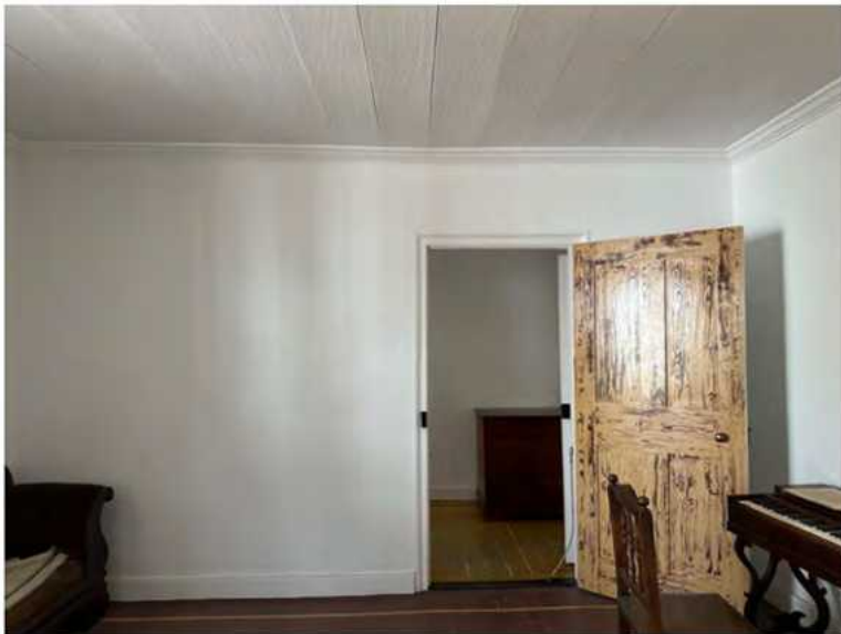
C: Room 101, looking E
