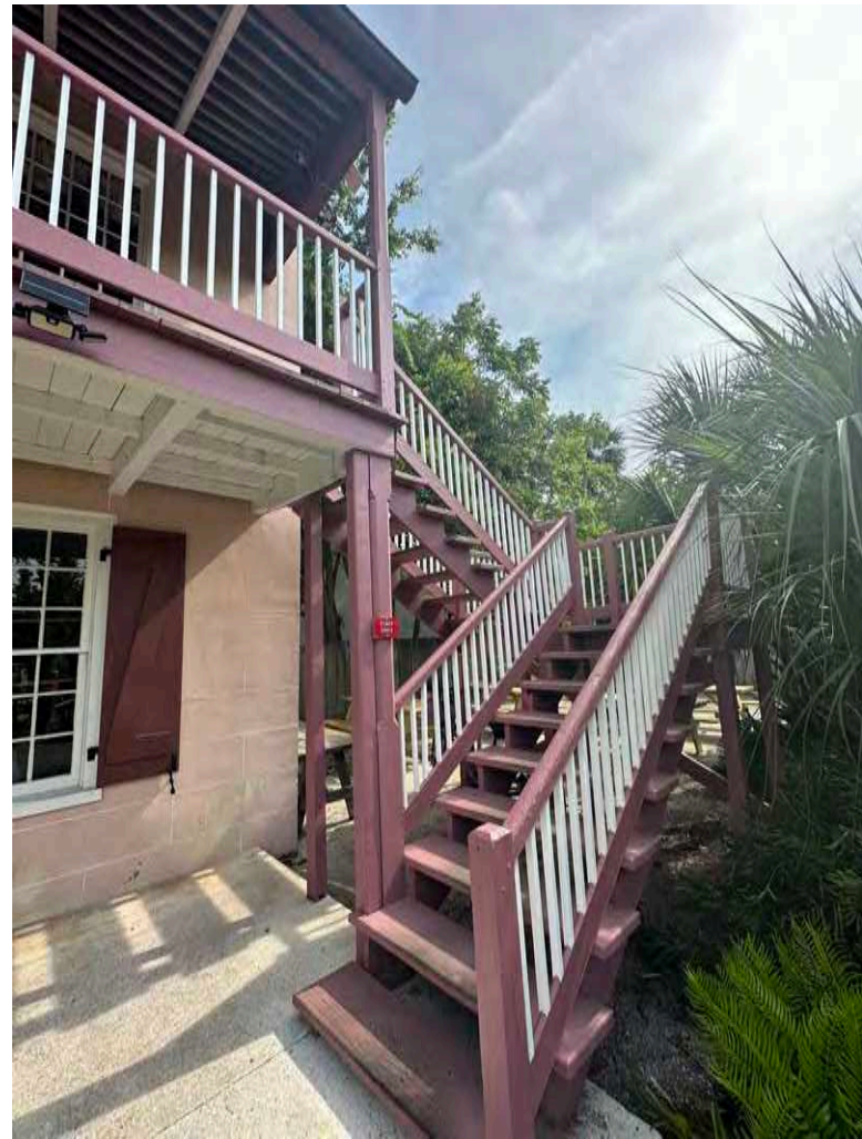
B: East Wing, loggia, looking NE
