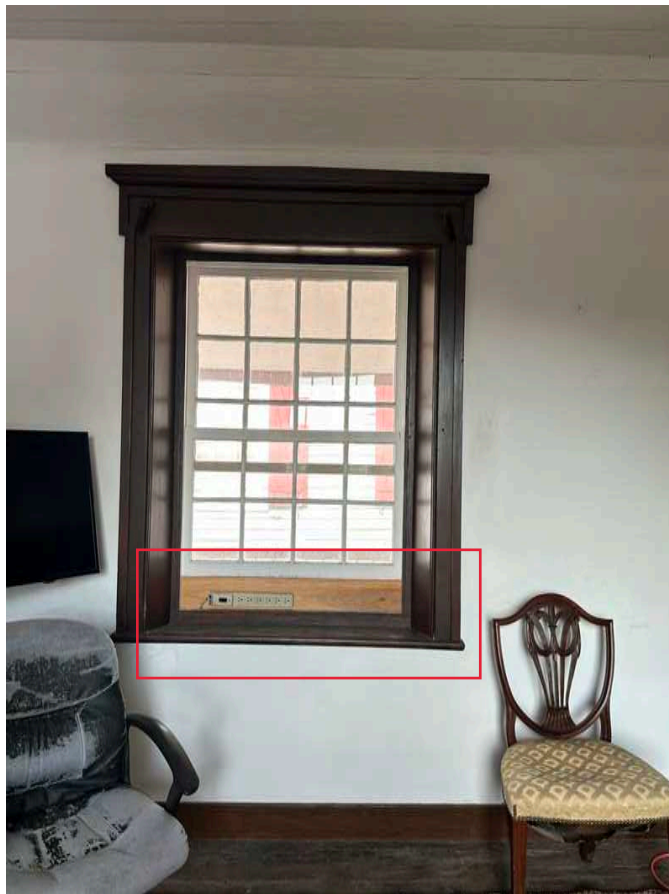
A: Room 201, looking W
