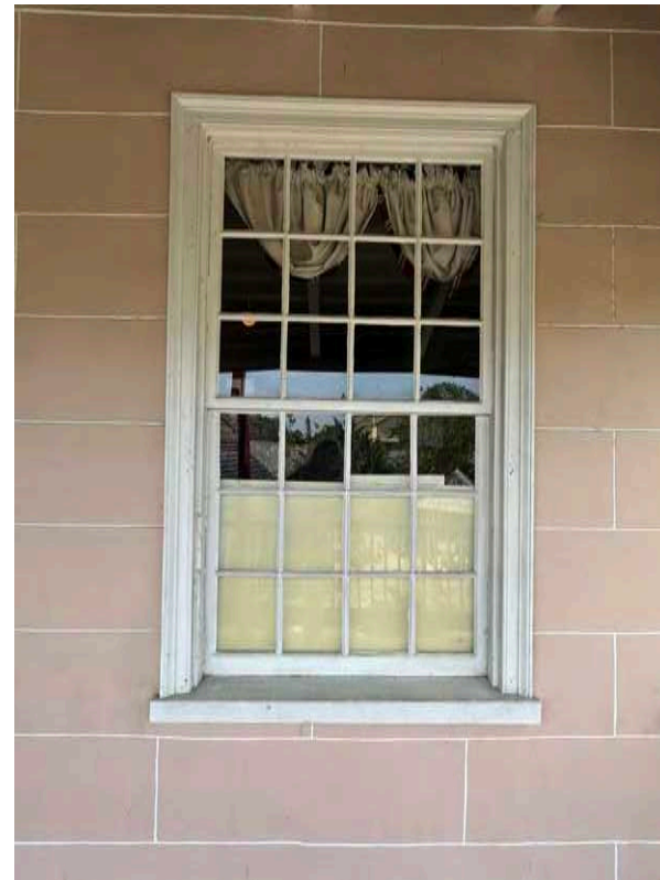
B: East Wing, window 2S1, looking N
