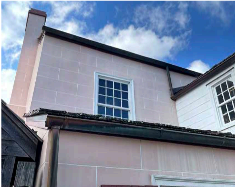
B: West Wing, E facade, looking NW
