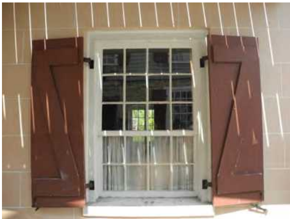
D: West Wing, W facade, looking E
