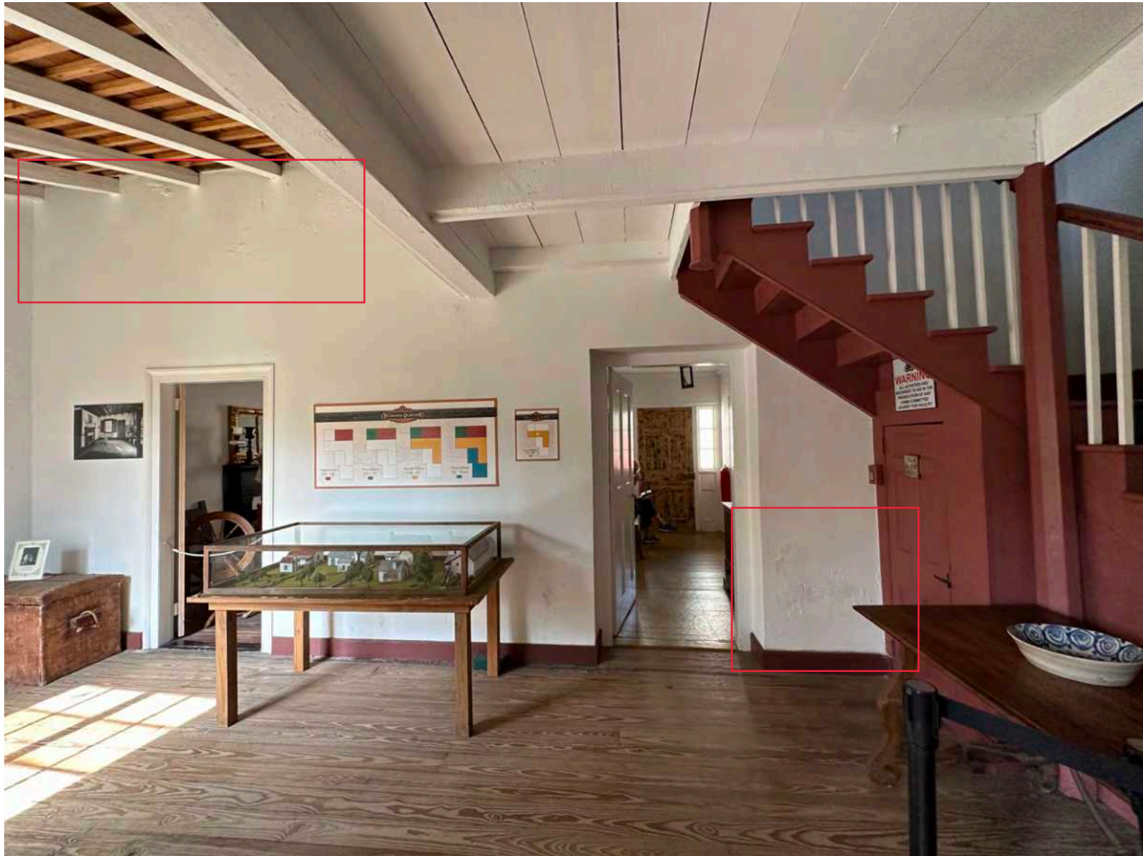
A: Rooms 104 and 105, looking SW
