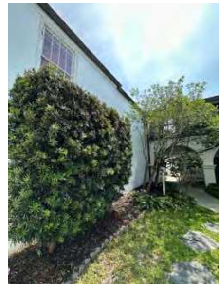
D: East Wing, N facade, looking E
