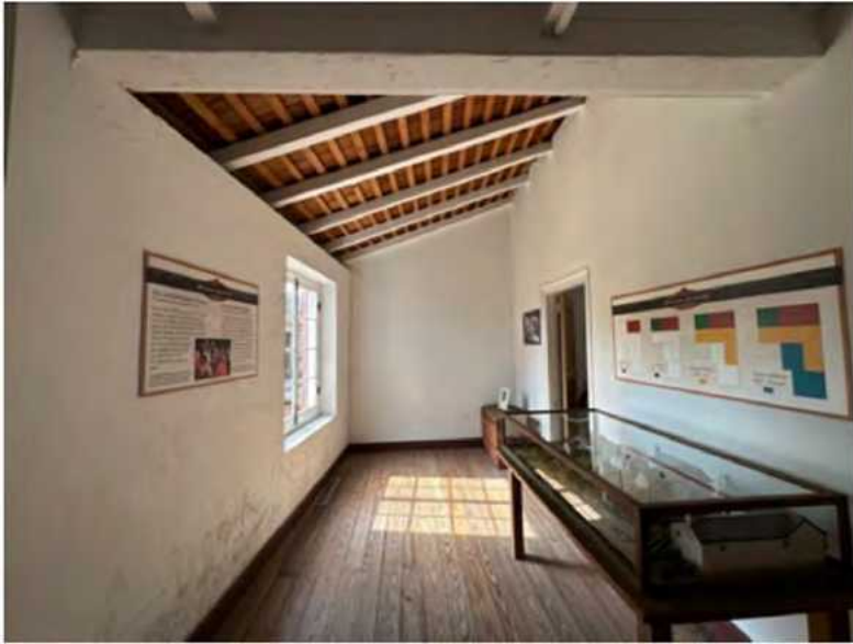
A: Room 104 looking S
