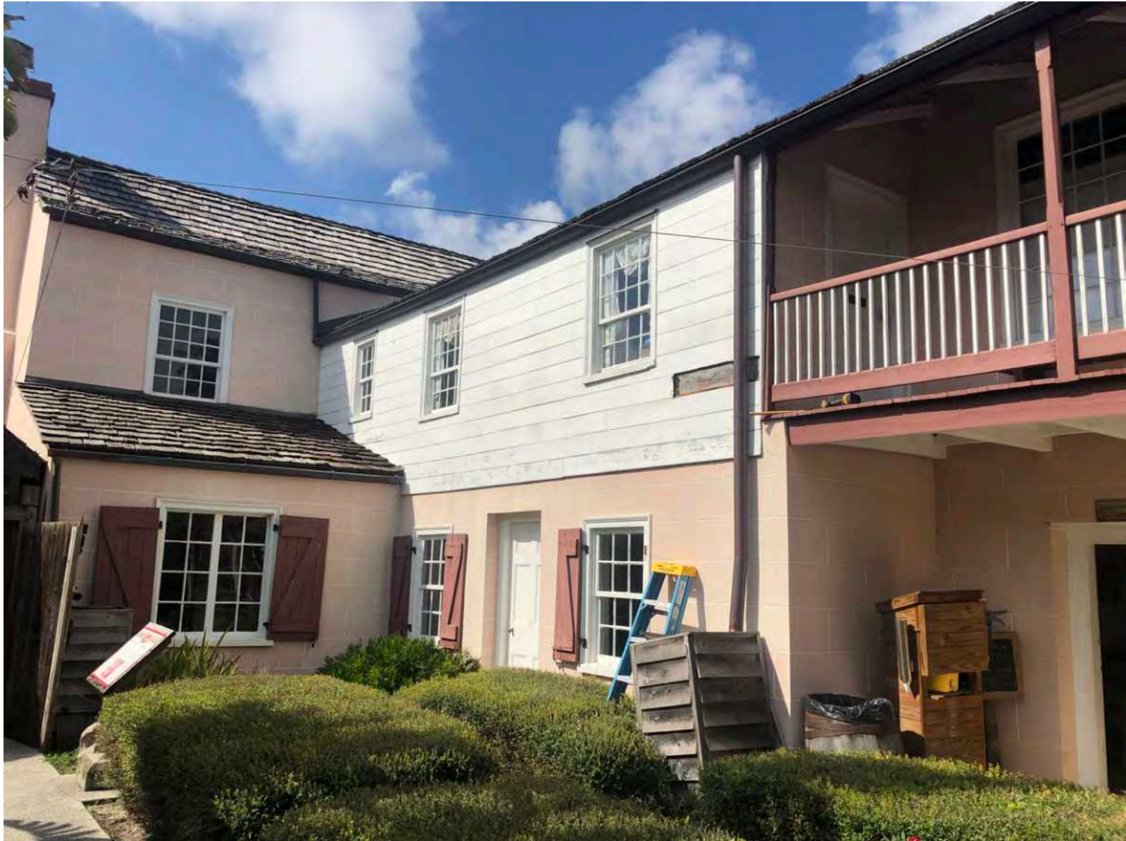
A: West Wing, roof's E slopes looking NW
