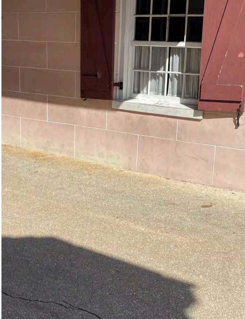
A: West Wing, W facade, looking NE
