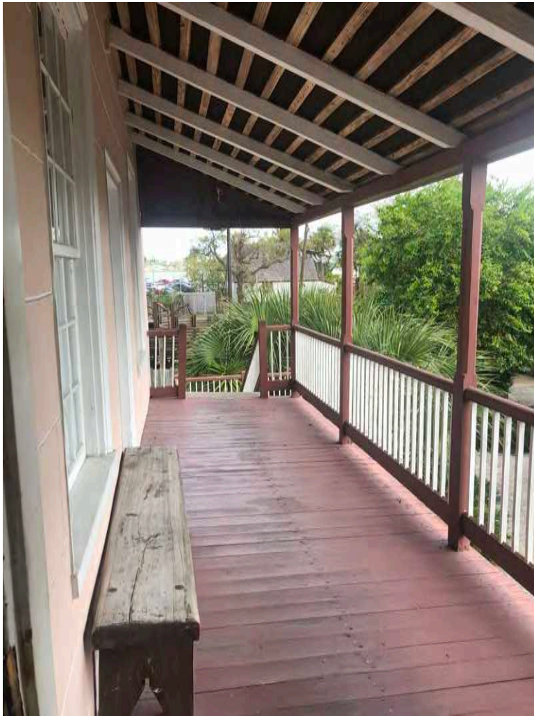
A: East Wing, loggia, looking E
