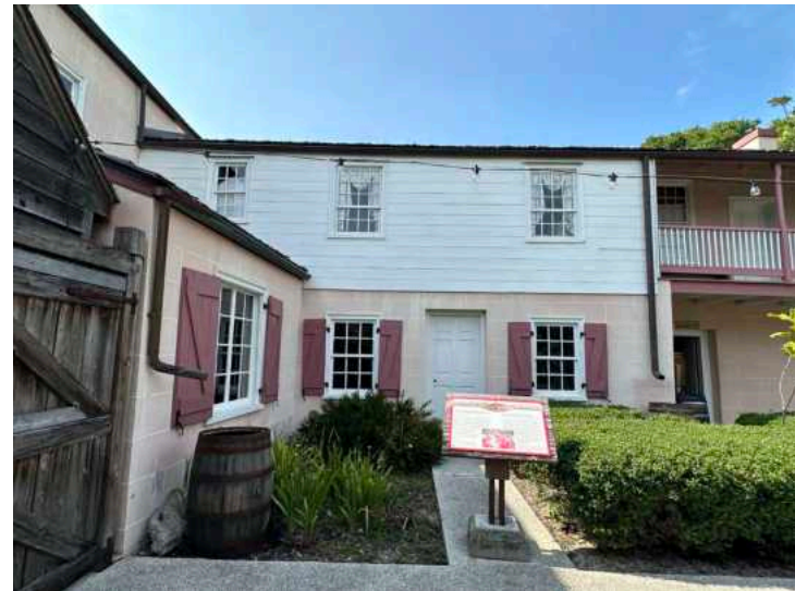
E: Concrete walkway, looking N
