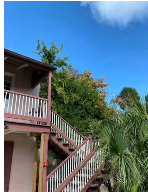
F: East Wing, Loggia, looking NE and up
