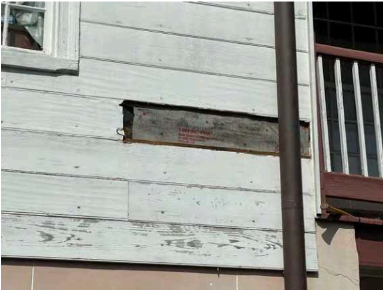
A: East Wing, S facade, looking NE, November 2022
