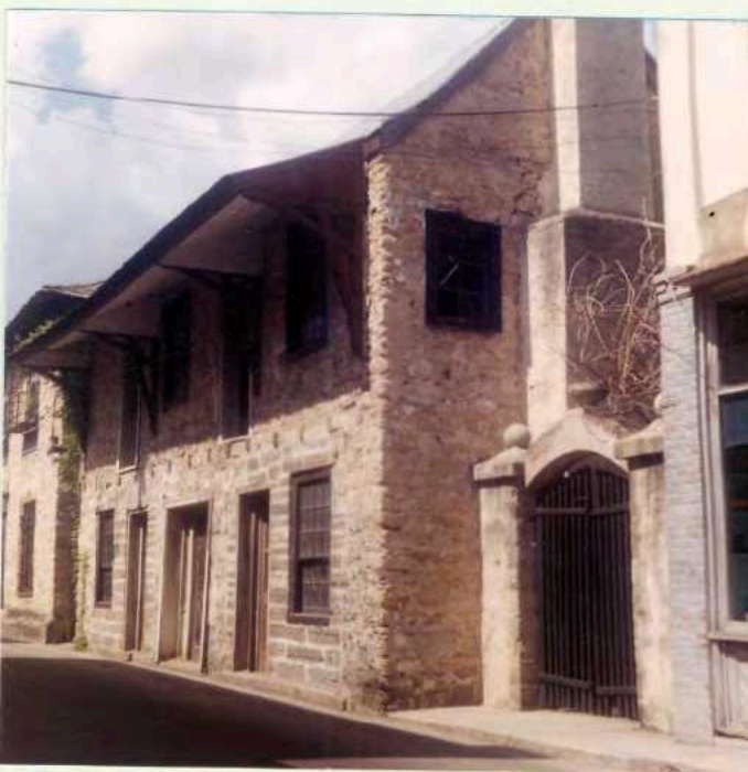
Figure 8 West Wing, west façade, prior to restoration of the balcony, looking Northeast, ca. 1958. https://original-ufdc.uflib.ufl.edu/USACH00551/00080/1x
