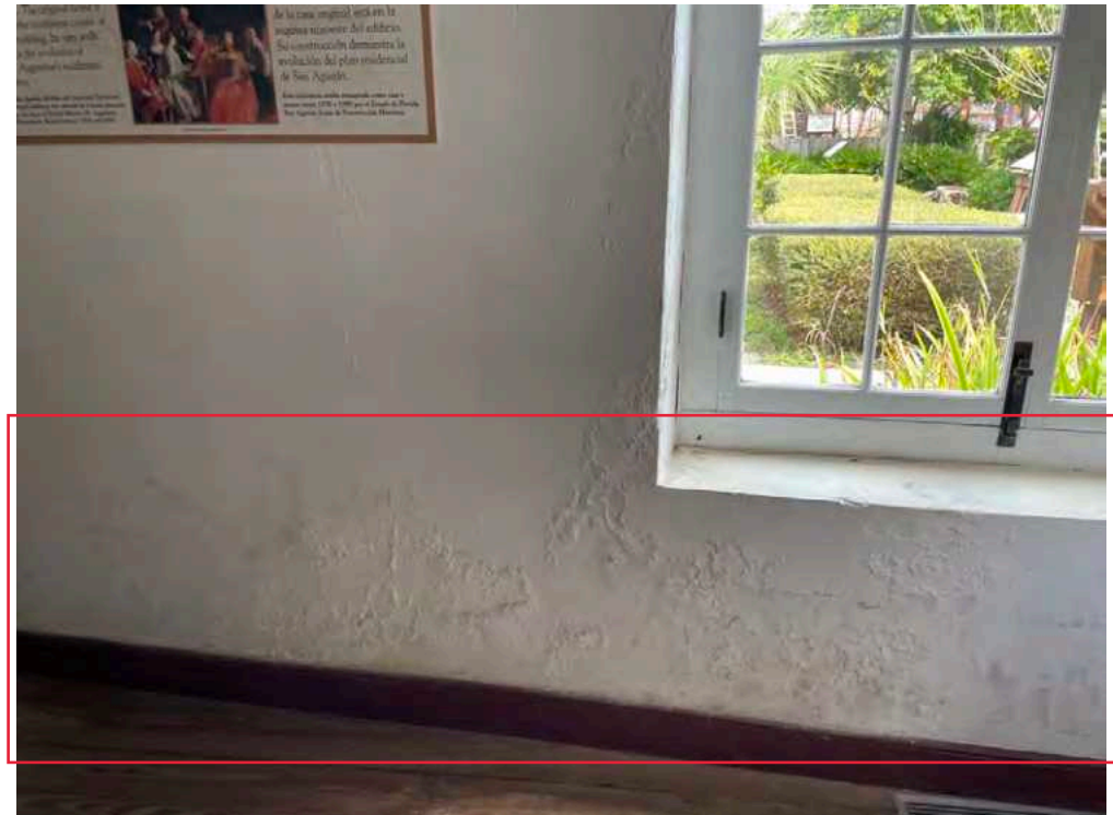
C: Rooms 104 and 105, looking E and down
