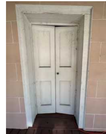
G: West Wing, W facade, looking E
