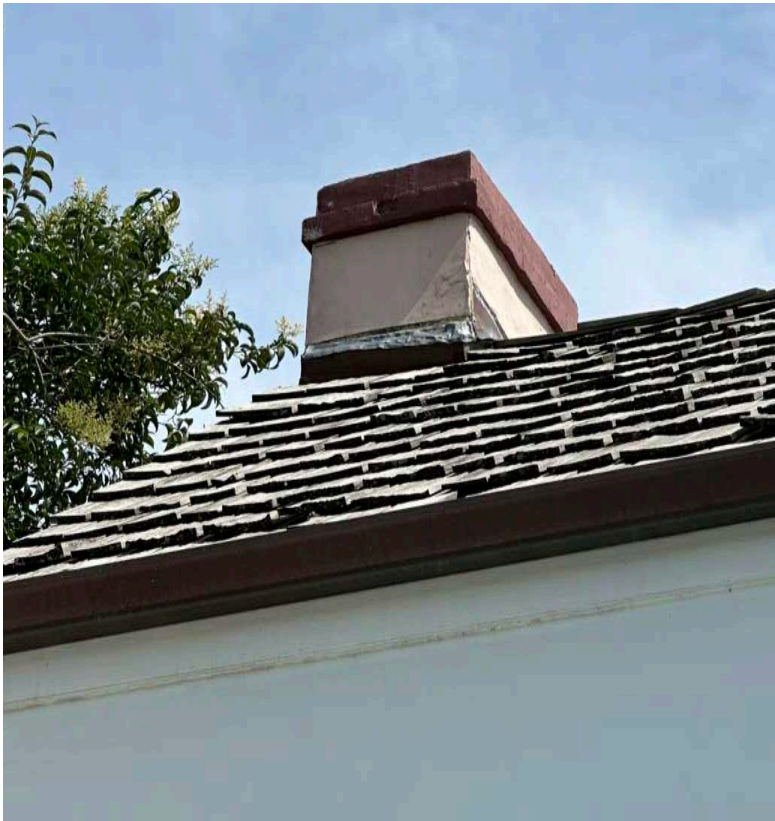
B: East Wing, roof's N slope, looking SE and up
