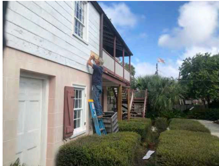
C: East Wing, S facade looking E
