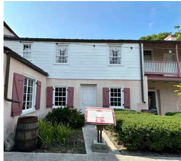
C: Door D13 East Wing, S facade, looking N
