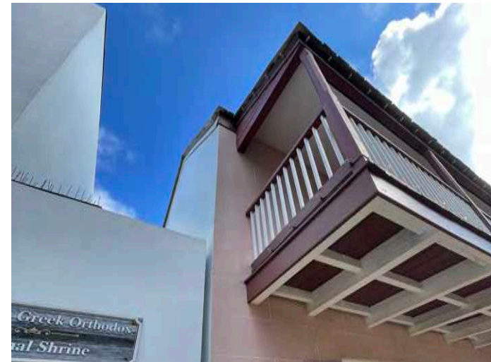
C: West Wing, Balcony, looking SE and up
