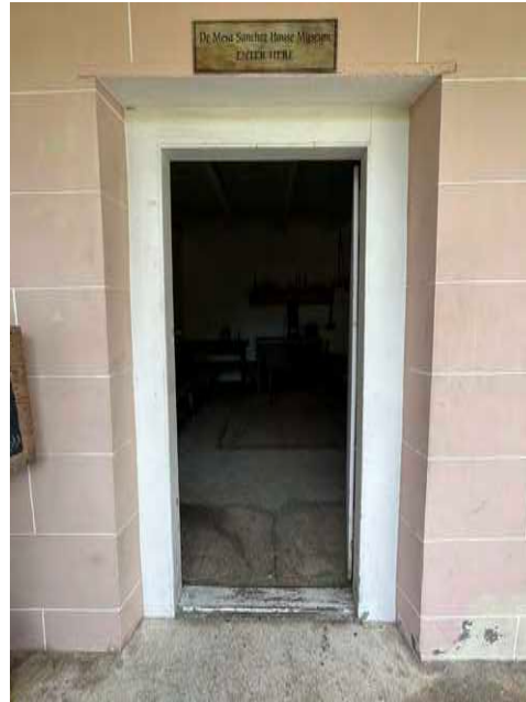
B: Door D11 East Wing, S facade, looking N
