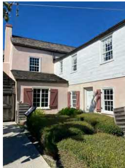
C: East Wing, S facade, looking NW
