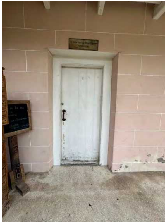
C: East Wing, S facade, door D11
