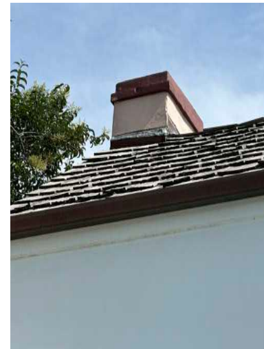
C: East Wing, N facade, looking S
