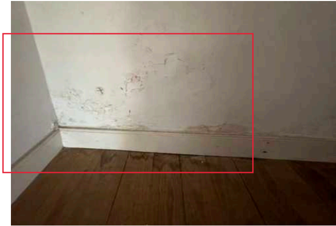
A: Room 108, looking NW
