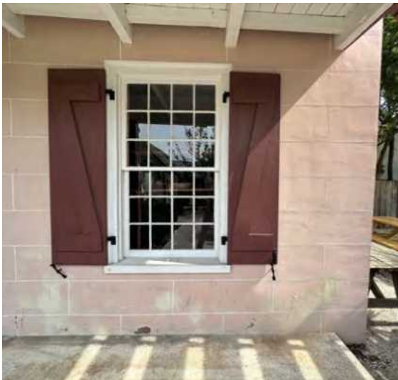
D: East Wing, Loggia, looking N
