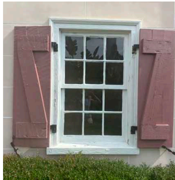
B: East Wing, window 1S2, looking N
