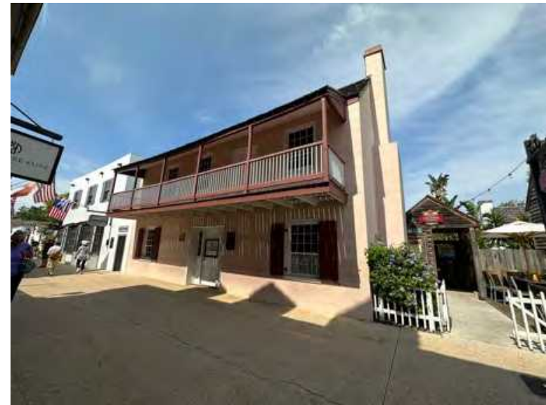
A: West Wing, W facade looking NE
