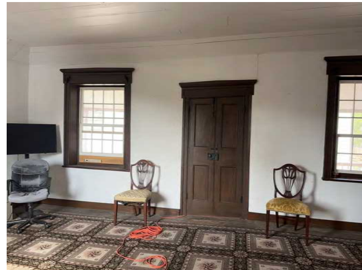
B: Room 201, W wall, looking SW
