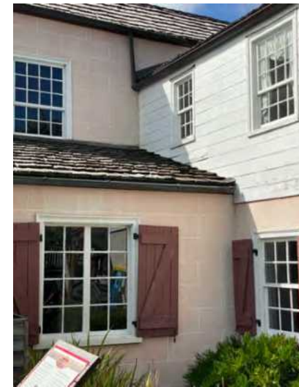
A: West wing, E facade, East Wing, S facade, looking NW
