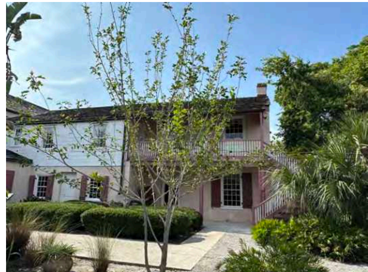
E: Concrete walkway, looking NW
