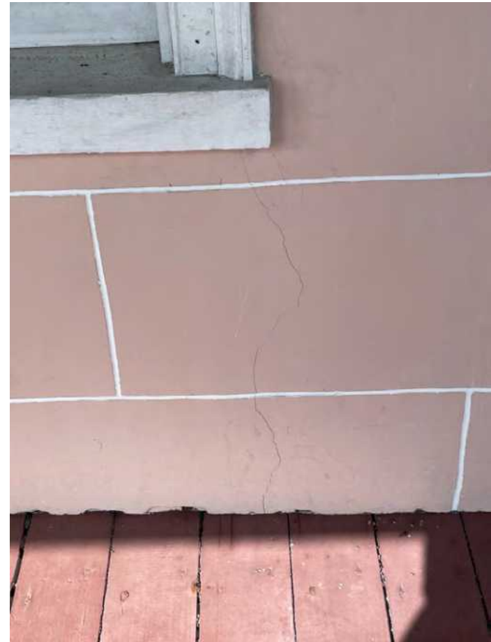
C: East Wing, S facade, looking N
