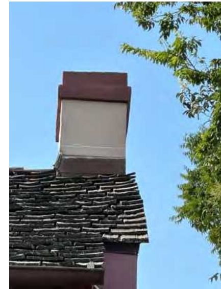
E: South Wing, S facade, looking N and up
