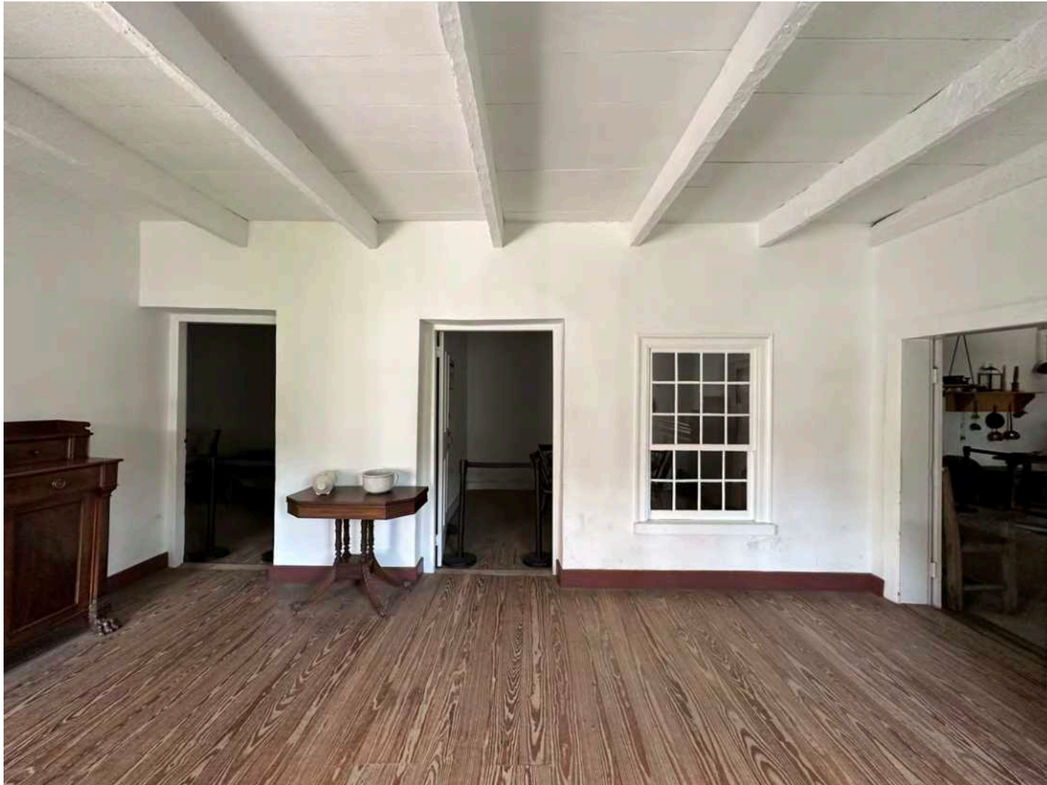
A: Room 107 looking N
