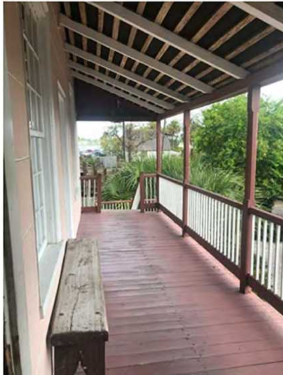
B: East Wing, Loggia, looking E
