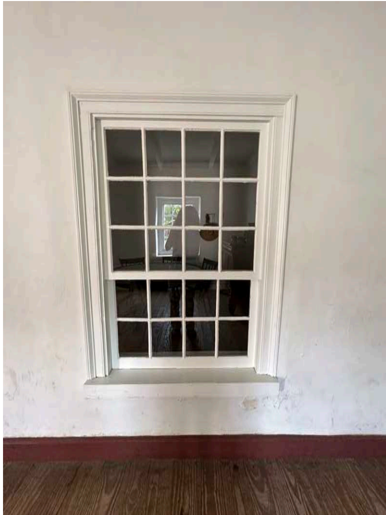
A: Window 111, looking N
