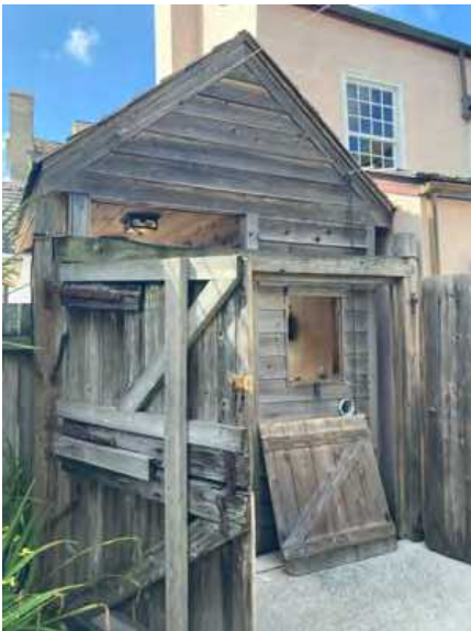
B: Auxiliary structure, looking NE
