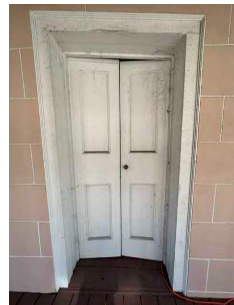
C: Door D14 West Wing, W facade, looking E
