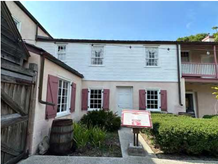
A: East Wing, S facade, looking N
