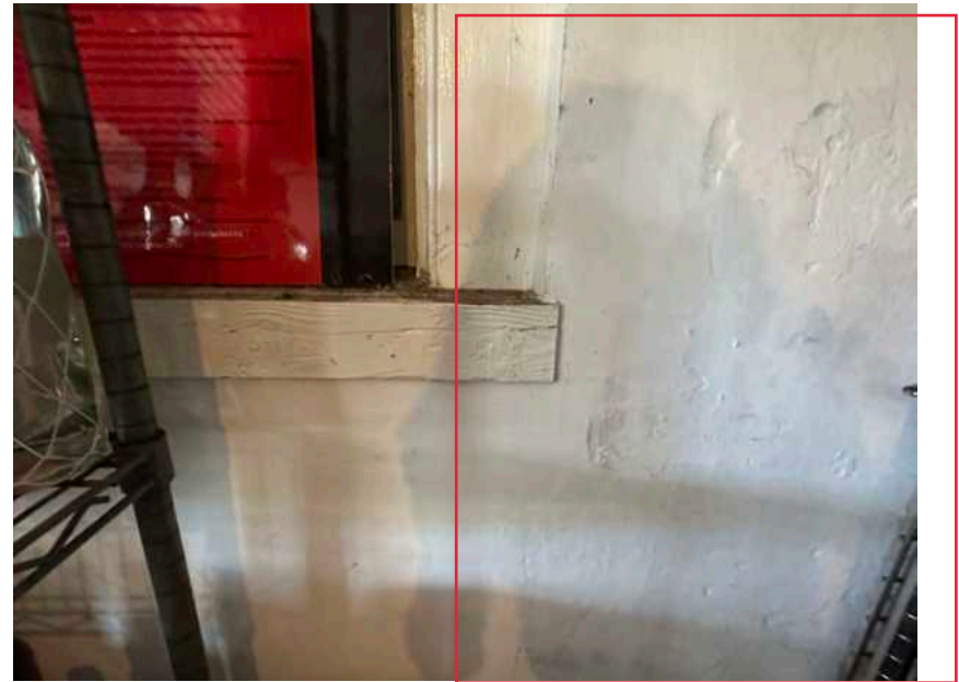
B: Room 210, window 2N1, looking N
