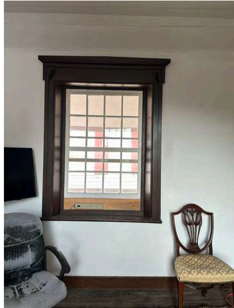
B: Window 2W1, looking W
