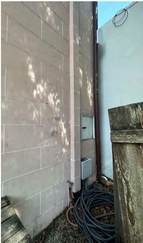
A: East Wing, east facade, looking NW
