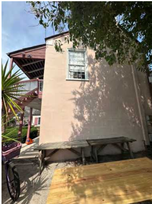
A: East Wing, S facade, looking NW
