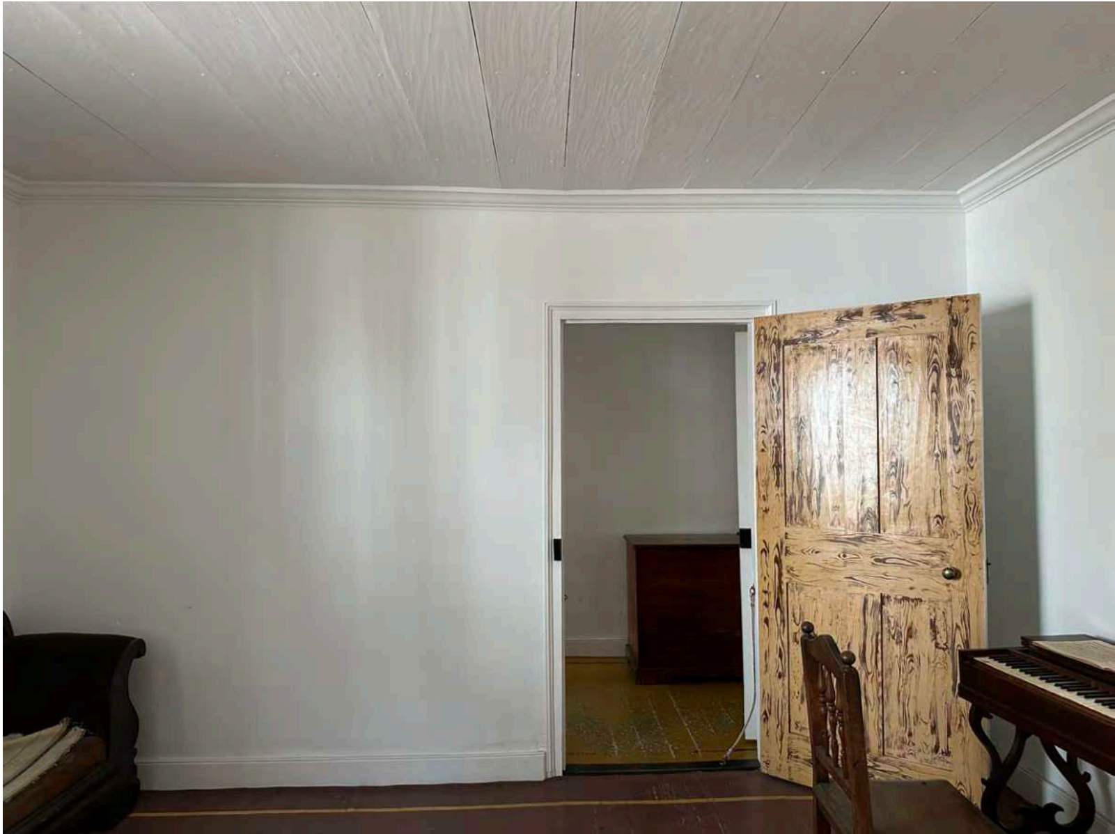
C: Door 2D, looking N
