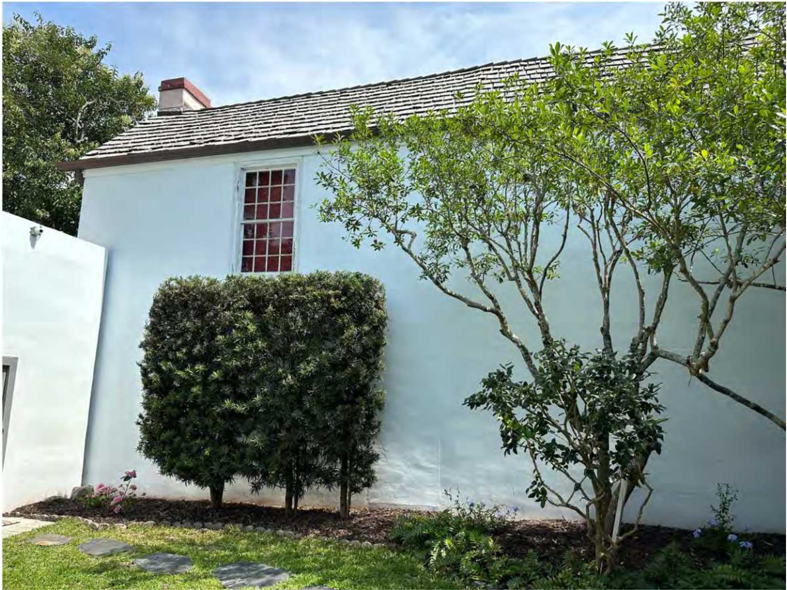
E: East Wing, N facade, looking SE
