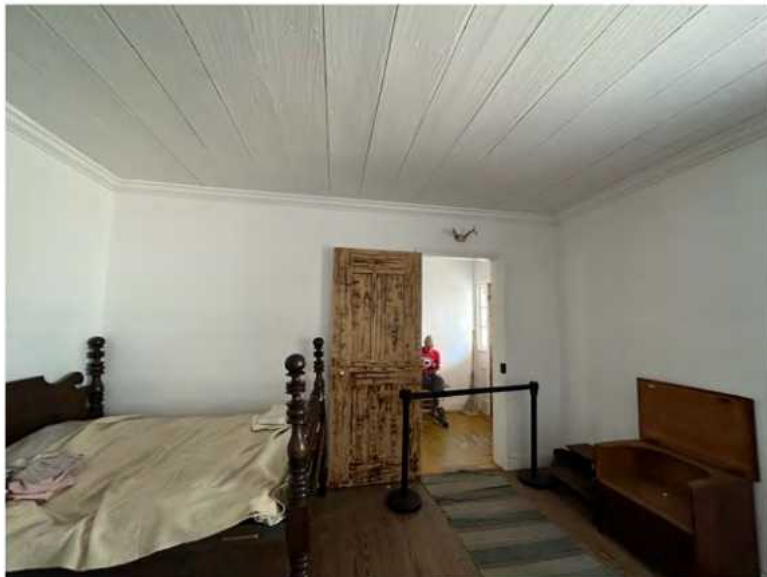
C: Room 103, looking SW
