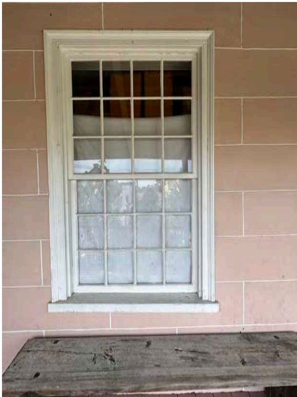
A: East Wing, window 2S2, looking N
