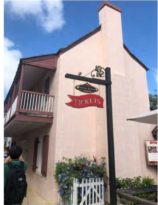
B: West Wing, S facade, looking NE
