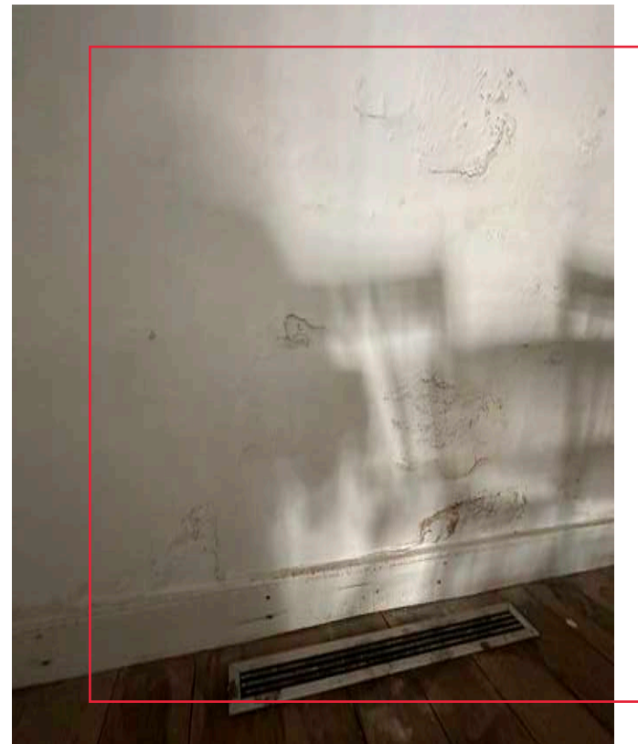
C: Room 108, looking NE
