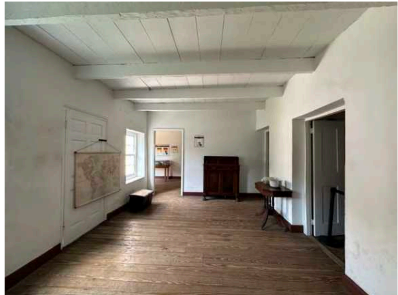
D: Room 107, looking W
