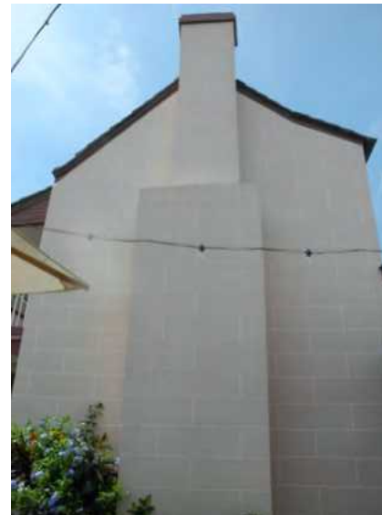
D: West Wing, S facade, looking N and up
