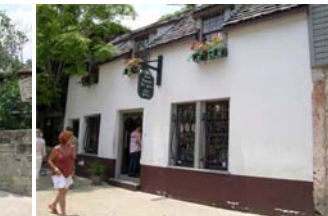
3903 Paredes Dodge House
